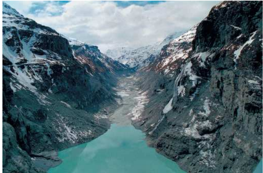
Mauvoisin reservoir: Empty reservoir with sedimentation
