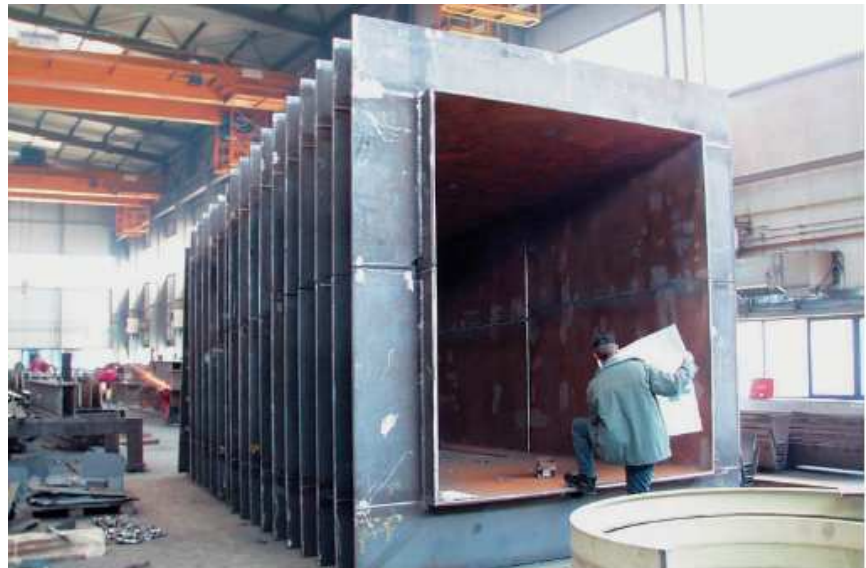
Workshop inspection of new steel liner
