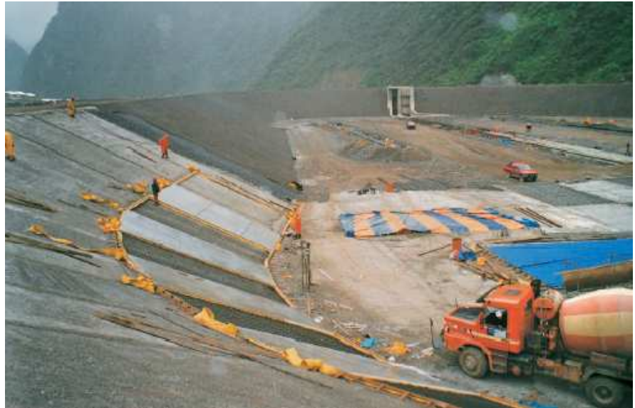
Regulation reservoir during construction
